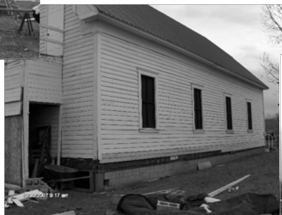
Upgrade to the Museum foundation and skirting
