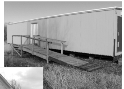
Storage Facility entrance added
