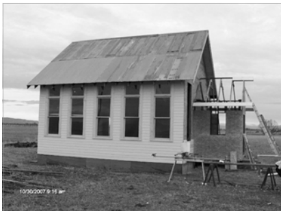
School House renovation begins!
